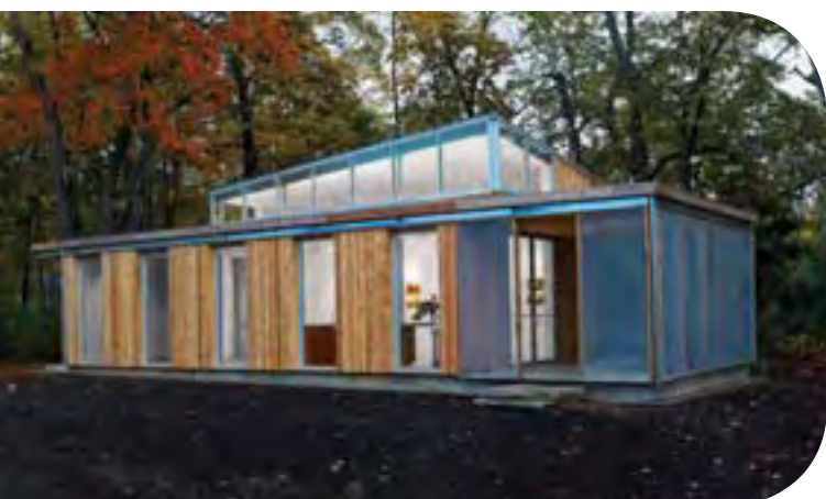
IIT students participate in the demolition of the original Meadow Studio under the supervision of Associate Professor Frank Flury [above center]. The new Meadow Studio opened last October [above].
